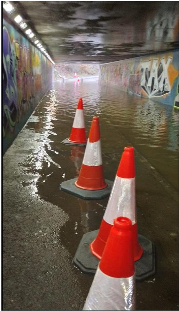
the A1(M) underpass subway to Hatfield
