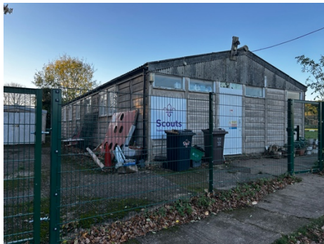
View of the Scout hut with new fencing
