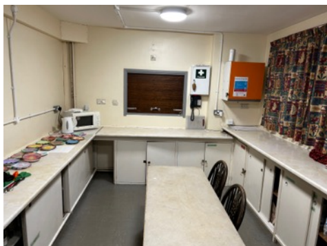
Kitchen fittings have not been modernized but is in reasonable condition
