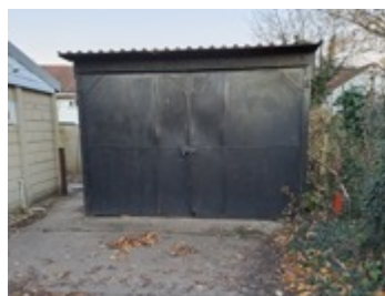
Lock up garage storage
