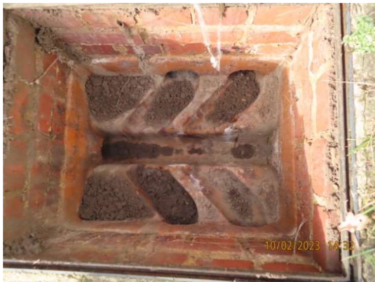
Interior of drainage inspection chamber with earth collected in branched outlets.
