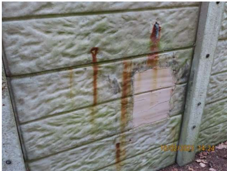
Infill to panel where boiler flue removed.
