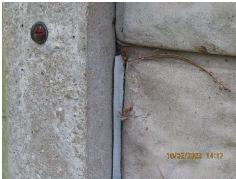
Mastic infill between panels and posts of concrete frame.
