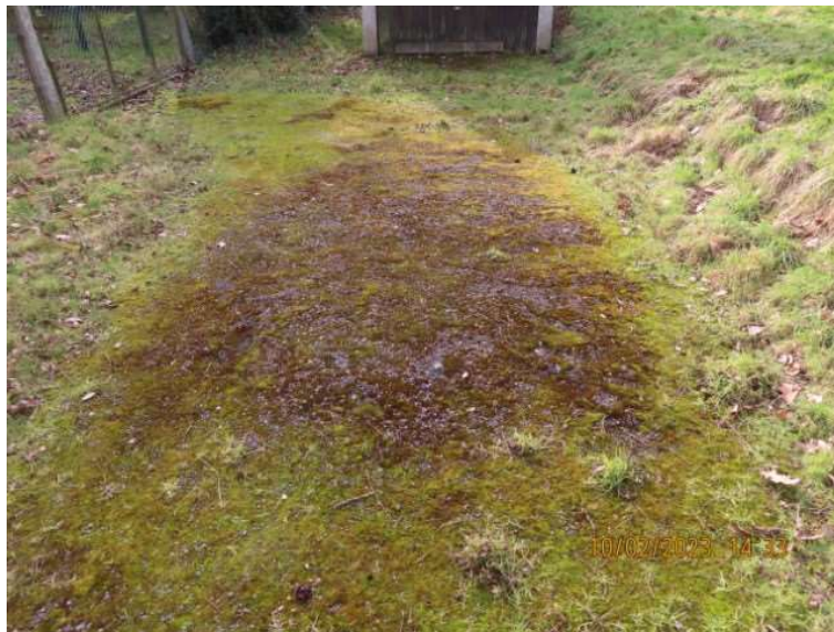
Overgrown moss and lichen on pathway.
