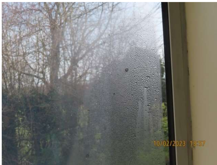
Interstitial condensation on perspex glazing.
