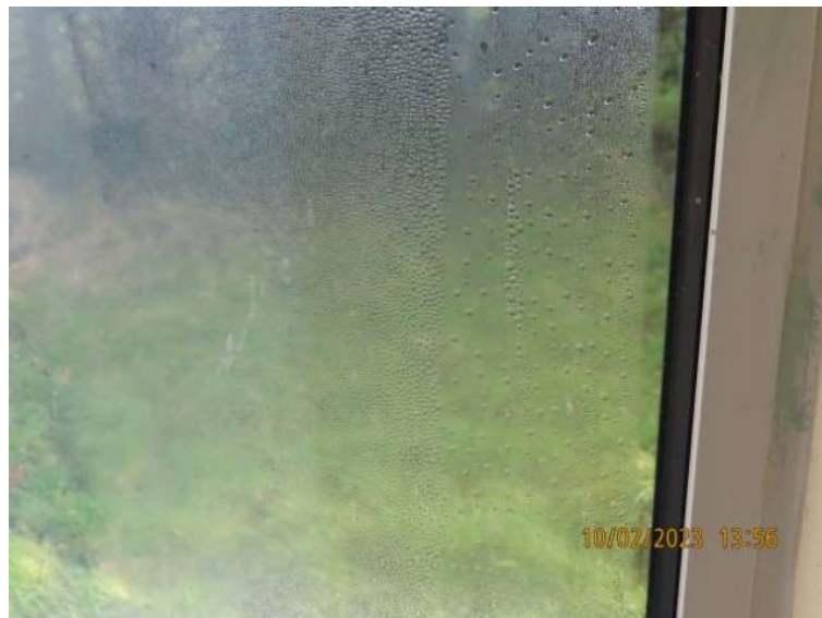
Interstitial condensation on perspex glazing.
